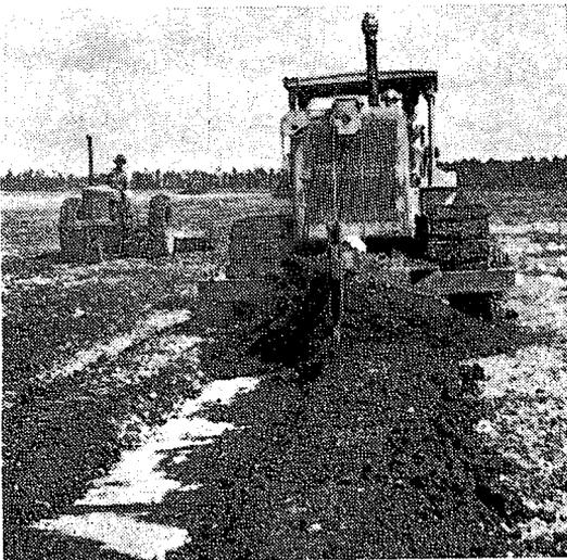
Figure 3. Final cut on rock soils of Dade County. The weight of the tractor helps crush cut rock.
